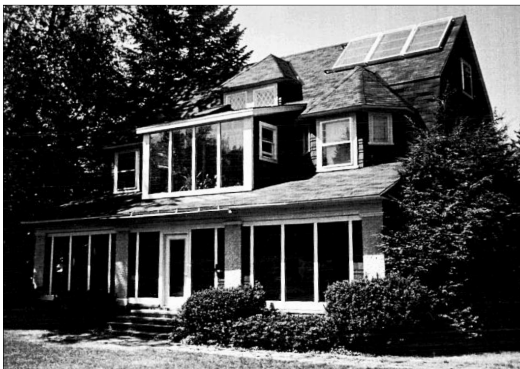
Homes such as this one use solar water heaters to supply most of the hot-water needs for the household.
