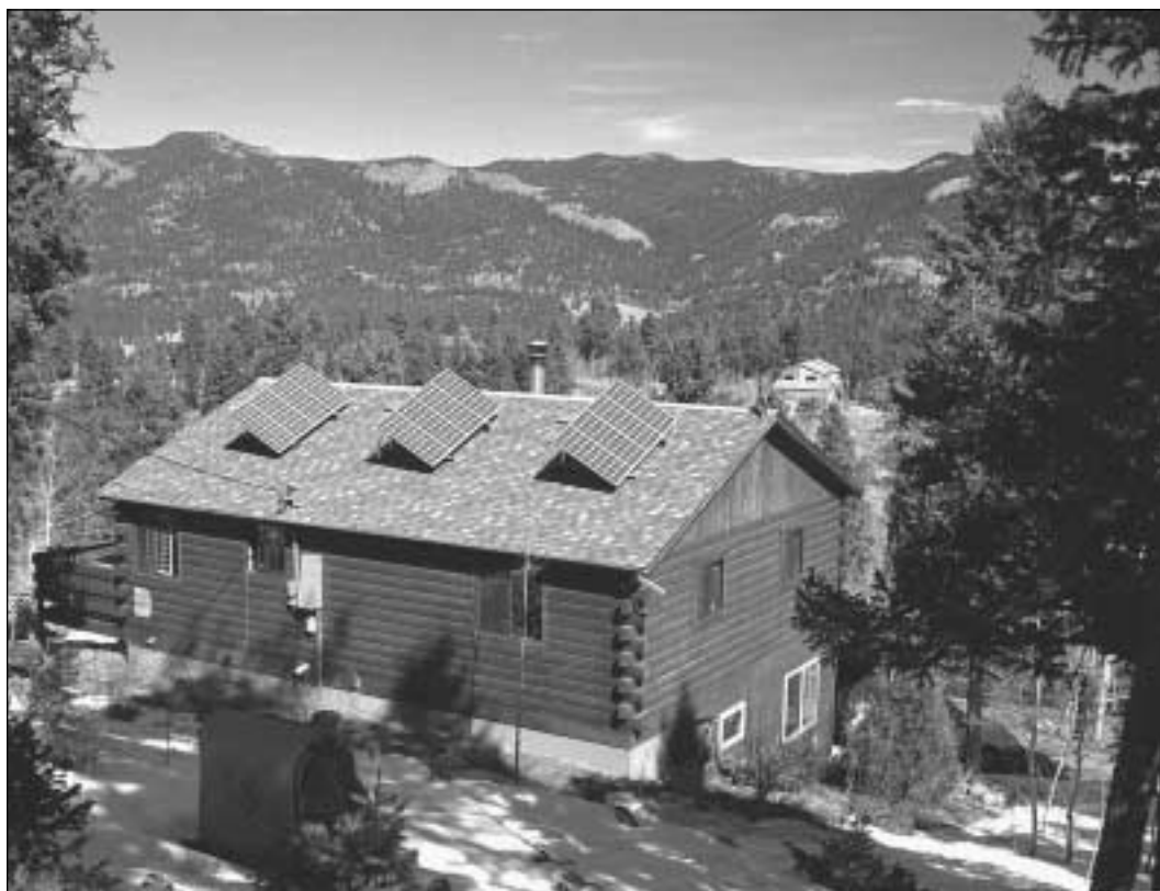
Terry Schuyler, NREL/PIX07679
