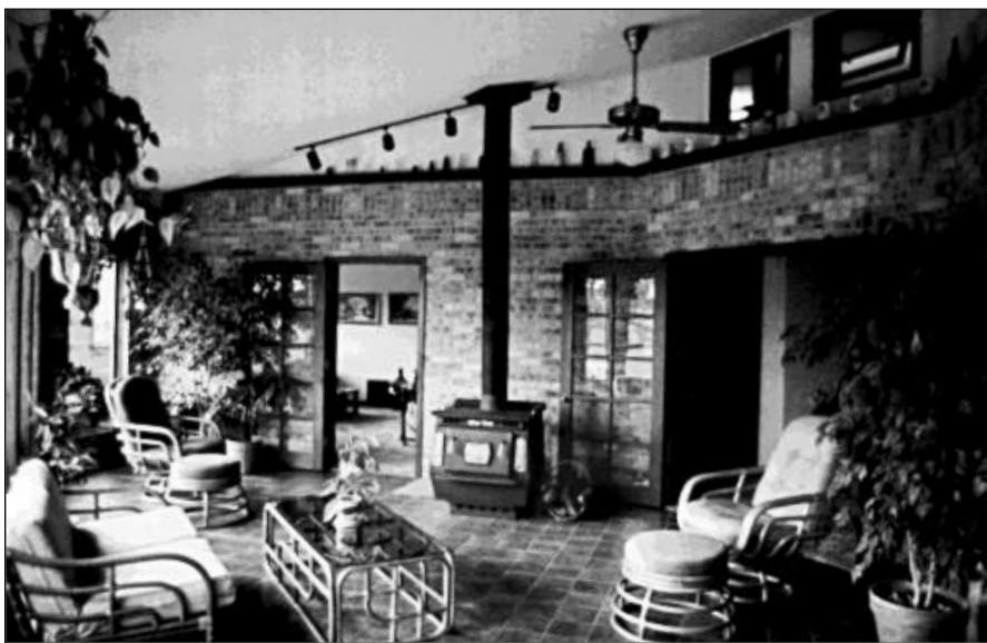
Tile floors and masonry walls provide thermal mass to store solar heat. Doors between sunspaces and other living areas can be opened to allow warm air to circulate.
