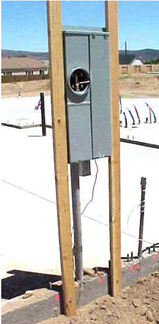
Figure 5 Semiflush Panel Mounting Using 2''x4'' Stud Framing
