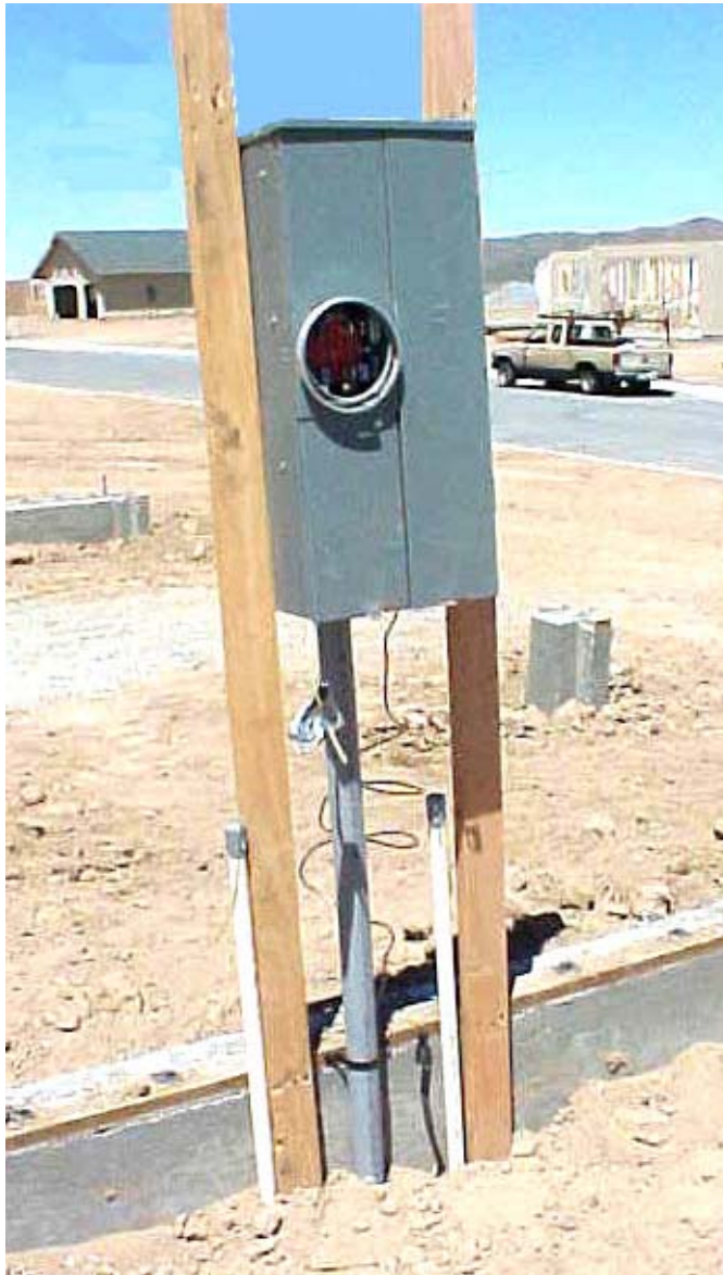
Figure 2 Surface Mount Panel w/ 2"x4" Stud Framing
