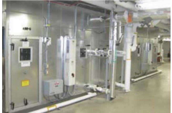
Large handling units benefit from variable speed drives
