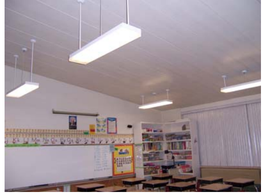
T8 Fluorescent Retrofit
