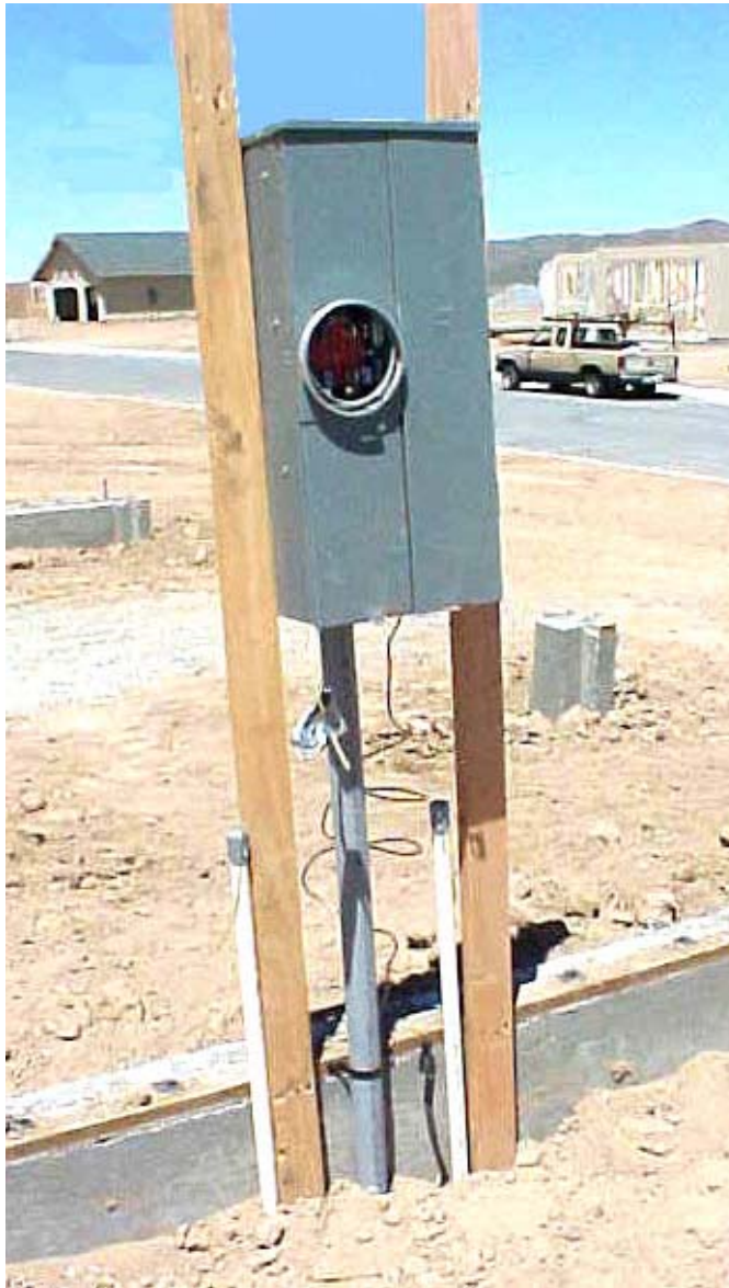
Figure 2 Surface Mount Panel w/ 2"x4" Stud Framing
