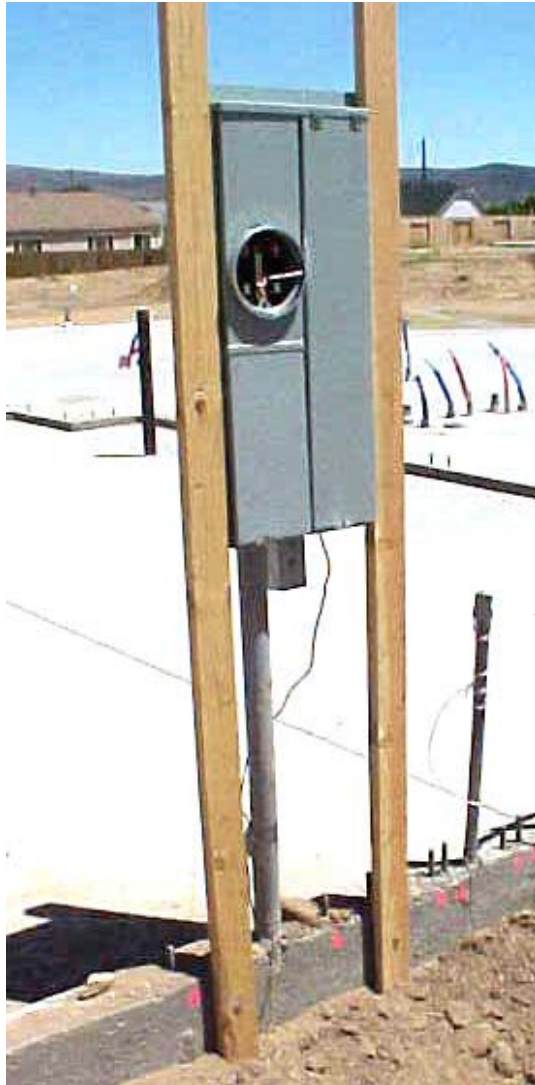
Figure 5 Semiflush Panel Mounting Using 2''x4'' Stud Framing
