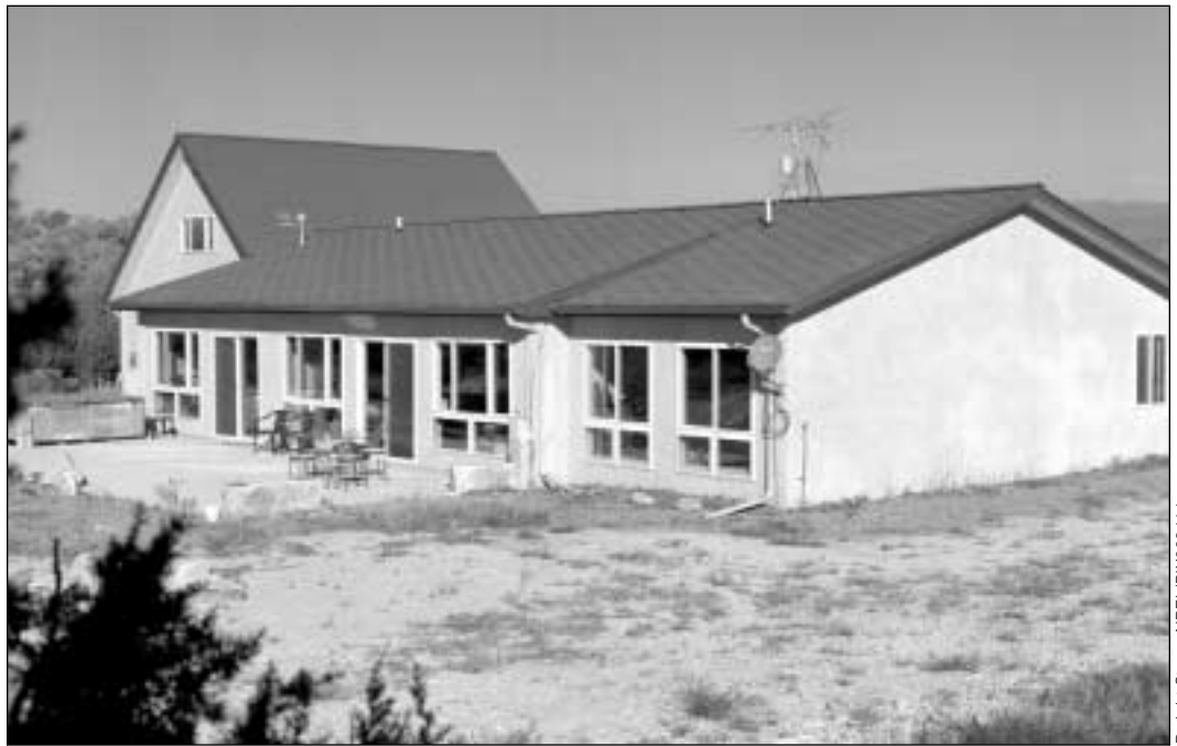
This passive solar home in Pueblo, Colorado — made from concrete forms, a high thermal mass material — only cost about 10 percent more to build than similar, conventional homes in the area.
