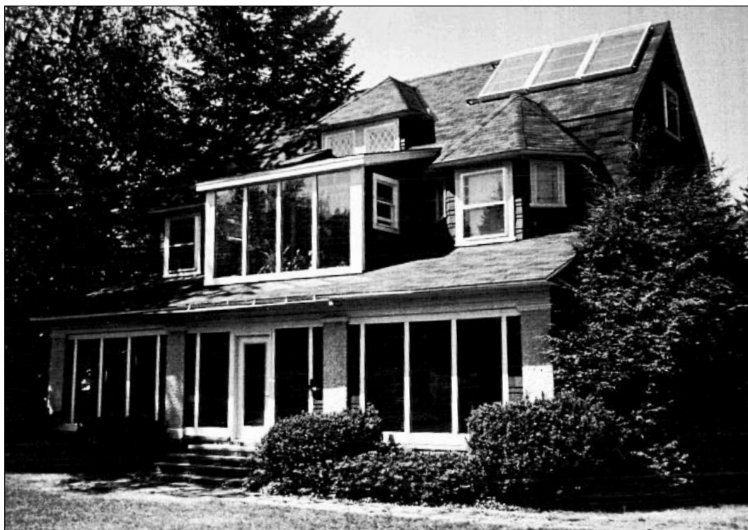
Homes such as this one use solar water heaters to supply most of the hot-water needs for the household.
