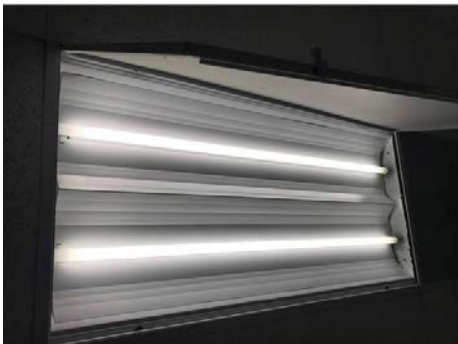
2x4 troffers in the main area with 2 T8 lamps each
