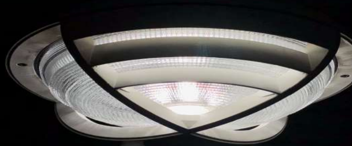
Retrofitted Parking Garage Fixtures
