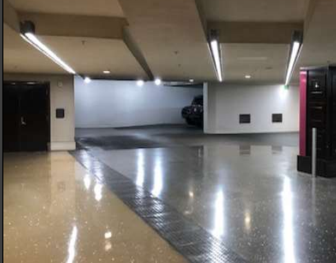
Existing Parking Garage Fixtures
